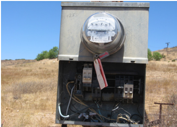
Tampering with the electrical meter can lead to fire, injury, or death
