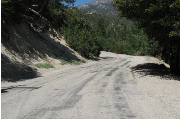
This area had a serious cement spillage
