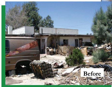
Structure that was abated in Thousand Palms
